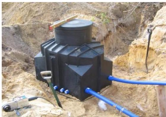
Photo 5 Collector well of the geothermal energy
