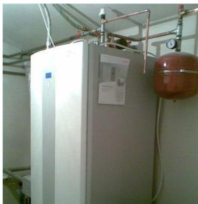
Photo 6 DHP-H 16 heat pump installed in the house
