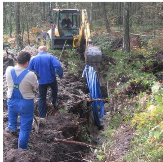
Photo 4 Horizontal heat collectors are installed in trenches
